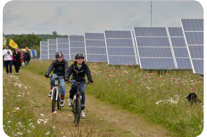
Westmill Solar Cooperative, UK. Courtesy of www.westmillsolar.coop .
