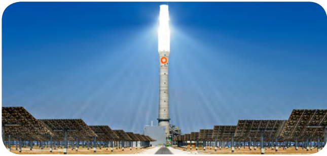
Gemasolar, Seville, Spain. Courtesy of www.torresolenergy.com
